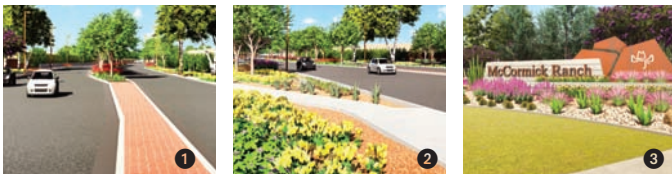
1) Median Renovation, 2) Right-of-Way Renovation, 3) Sign Renovation
